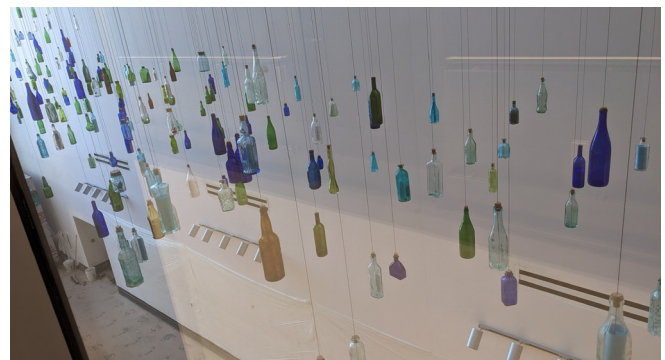
A close-up of the bottles during installation.
